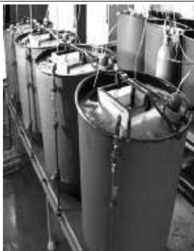
Figure 4. the tanks are circular with conical bottom. The upper diameter is about 70 cm, height 100 cm, and volume 250 L.
